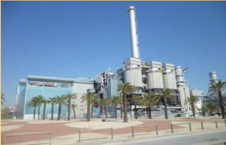
Barcelona, Tersa WTE Plant
